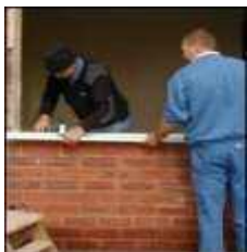
Check Aperture for Defects
