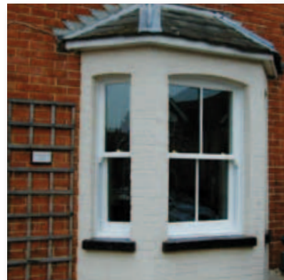
White VSS bay window with a single vertical astragal bar to the central window
