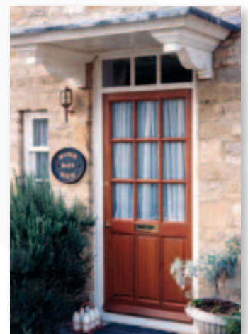
Front door with a storey frame and vertical bars aligning with the bars in the door. The frame is white and the door is mahogany
