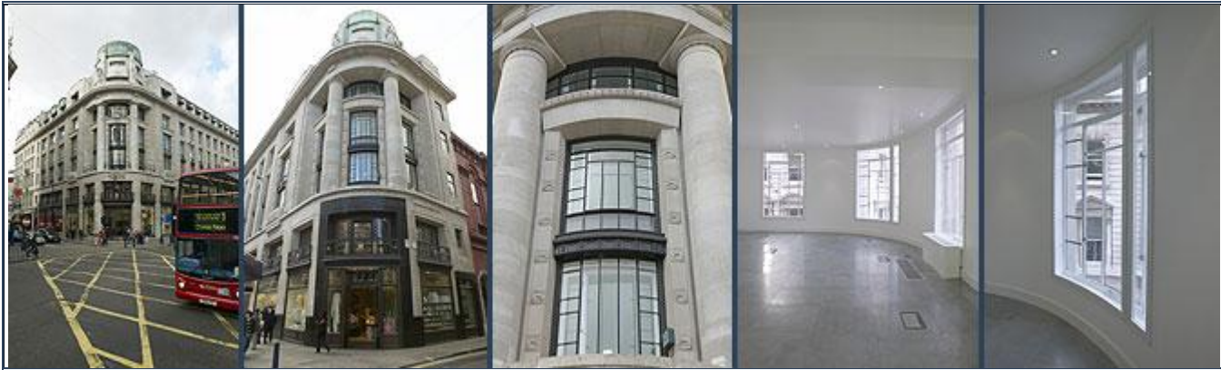
Primary Window Curved in the Plan Elevation - Secondary Glazing Curved & Paint Finished to Match & Fitted Unobtrusively
